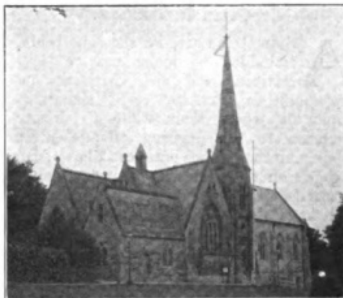
St. Luke's Church, Bath, fitted with Wireless Installation.
